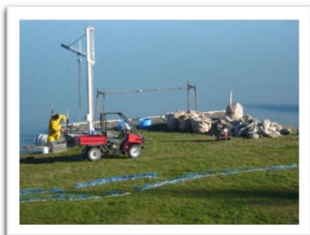
The picture on the left shows the lines of the dropper cords that attach the buoys to the lane wires. They were dunked in an approved detergent solution and then cleaned off with the water blaster. They were then strung out to dry. The amount of Didymo on the cords was quite amazing and the way it worked its way into the cord made it very difficult to remove. This may necessitate a change from cord to stainless steel wire.
