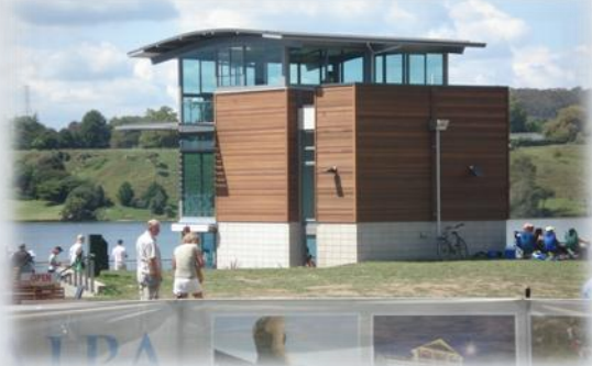
The New Finish Tower
